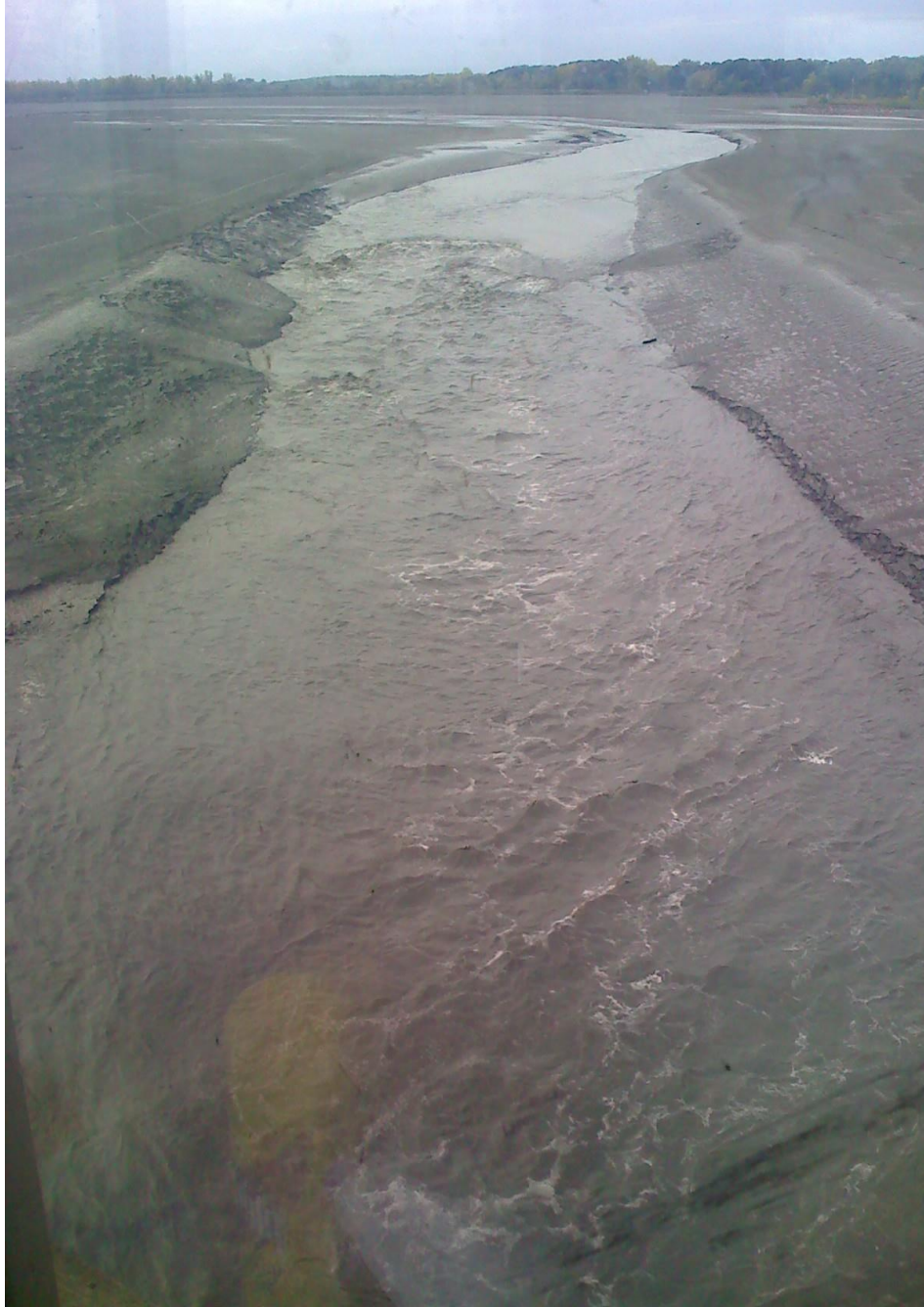
Flushing of the Assiniboine River Channel, upstream of the dam. The silt and sand shown on the left side of photo to be removed in early 2012.
