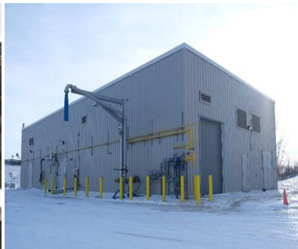
New Pre-treatment Building
