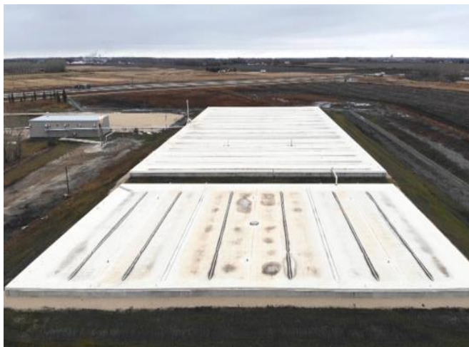
New LRAR and Burn Out Basin
