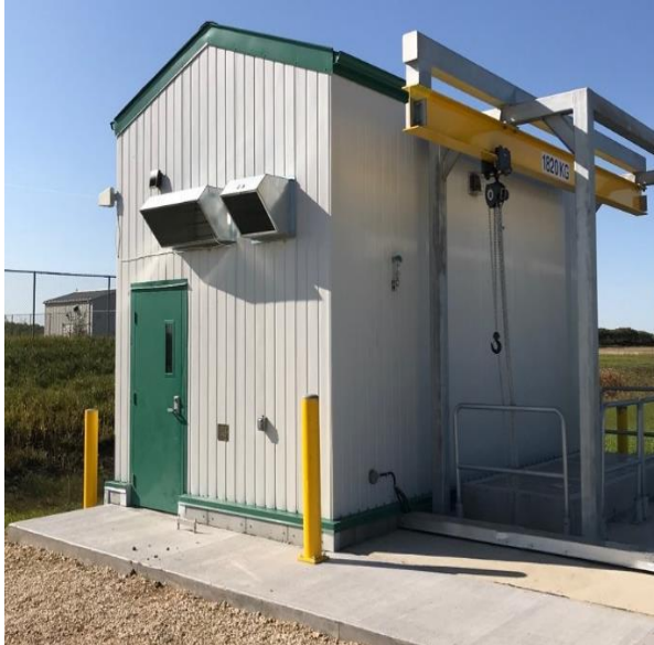
Poplar Bluff Lift Station- Exterior
