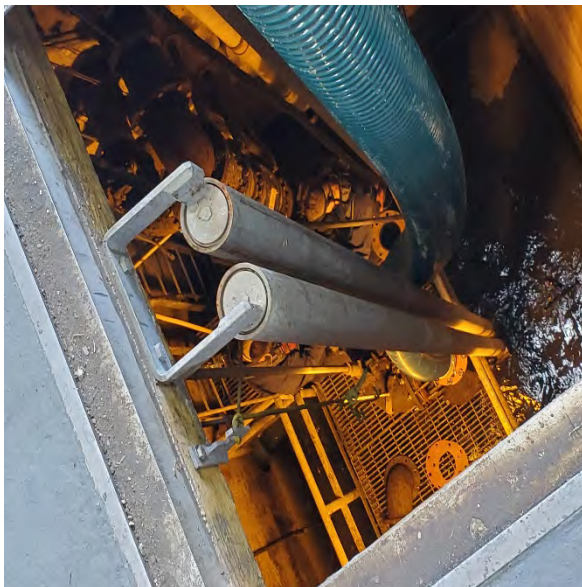
Staff working at Bridge Road Lift Station
